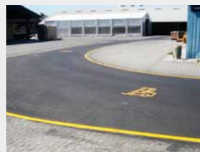
SAFE TRUCK-DRIVING New surface with yellow markings makes truck-driving safe at the Troldekt factory, Troldehede.
