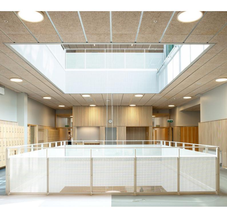
Troldtekt has developed the solution with visible longitudinal T-profiles in collaboration with JJW Arkitekter for the Sluseholmen School in Copenhagen. Therefore, we also refer to the solution as the "SLUS ceiling".
