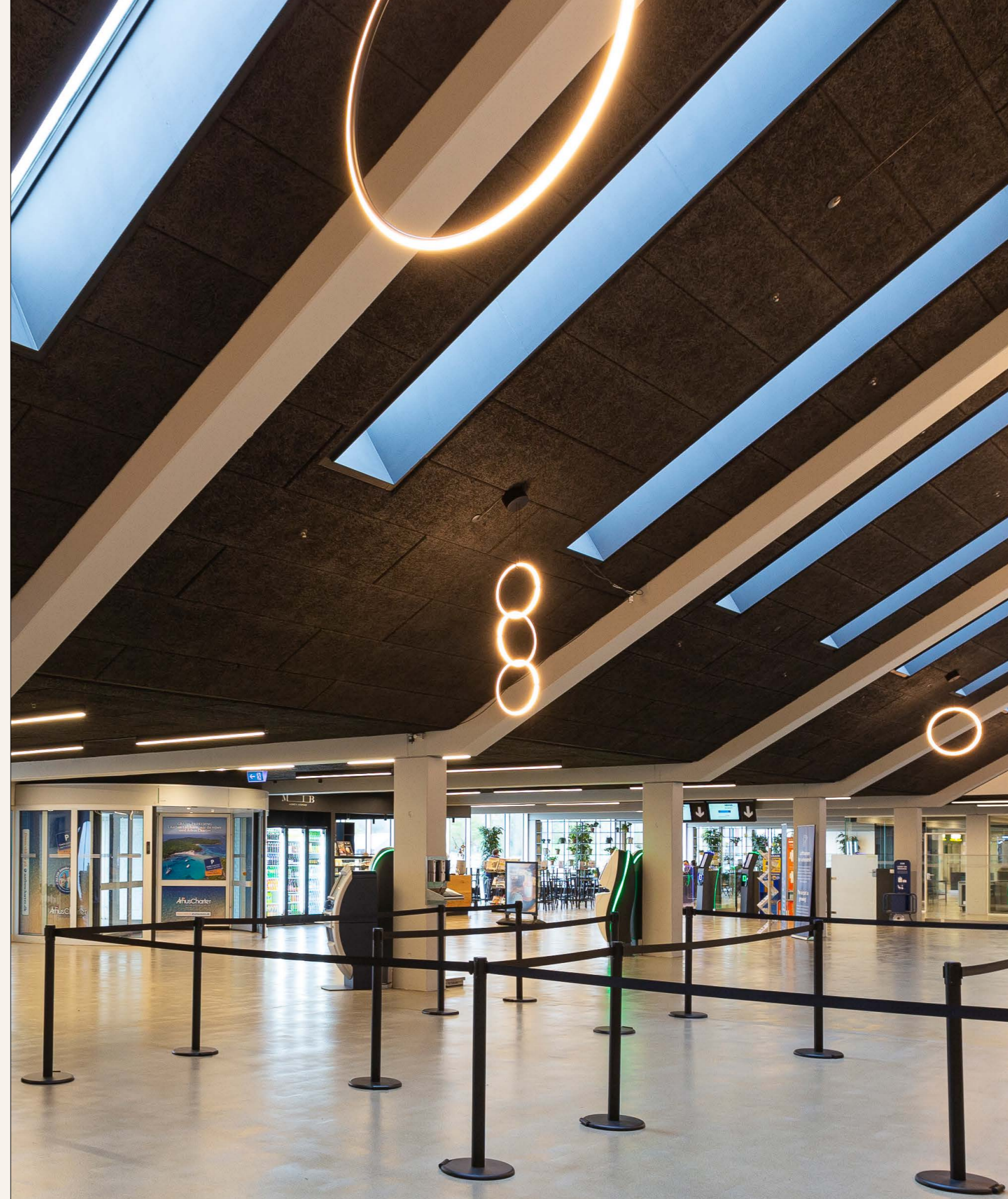
Trolldtekt acoustic panels can be repainted multiple times without compromising their properties. Aarhus Airport has chosen to extend the lifespan of its Trolldtekt ceilings by painting them black during the refurbishment.
