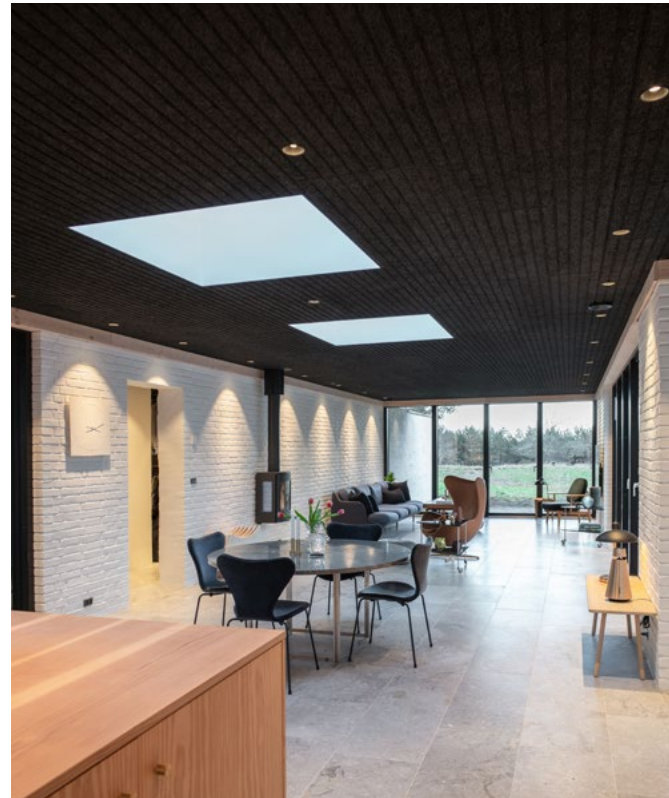
↑ A private home in which black-painted Troldekt v-line acoustic panels based on FUTURECEM have been chosen.
